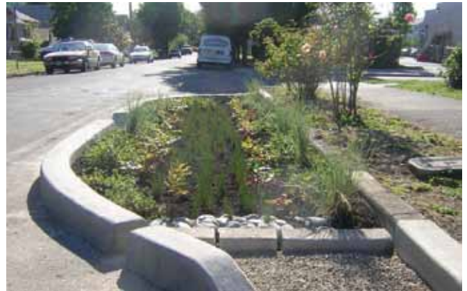
This example of a rain garden constructed at the street also serves as a traffic calming measure along a neighborhood roadway with higher speed traffic.
