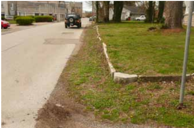
Examples of existing stormwater infrastructure in Cassville that do not adequately manage storm runoff.
