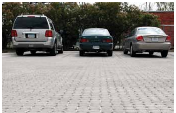
Permeable paving methods allow the movement of water around and through the paving material and into the soil. Such paving methods can be used for roads, parking lots, driveways and walkways in residential and commercial areas to help minimize the quantity of stormwater runoff.
