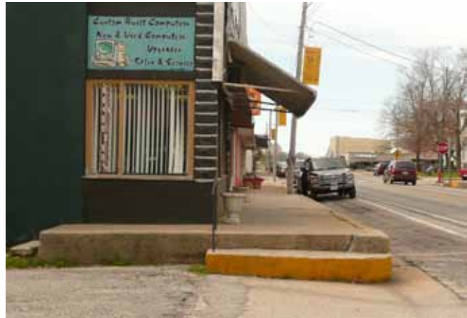
Steps up to sidewalks and high curbs are hazards to pedestrians and do not meet ADA requirements.
