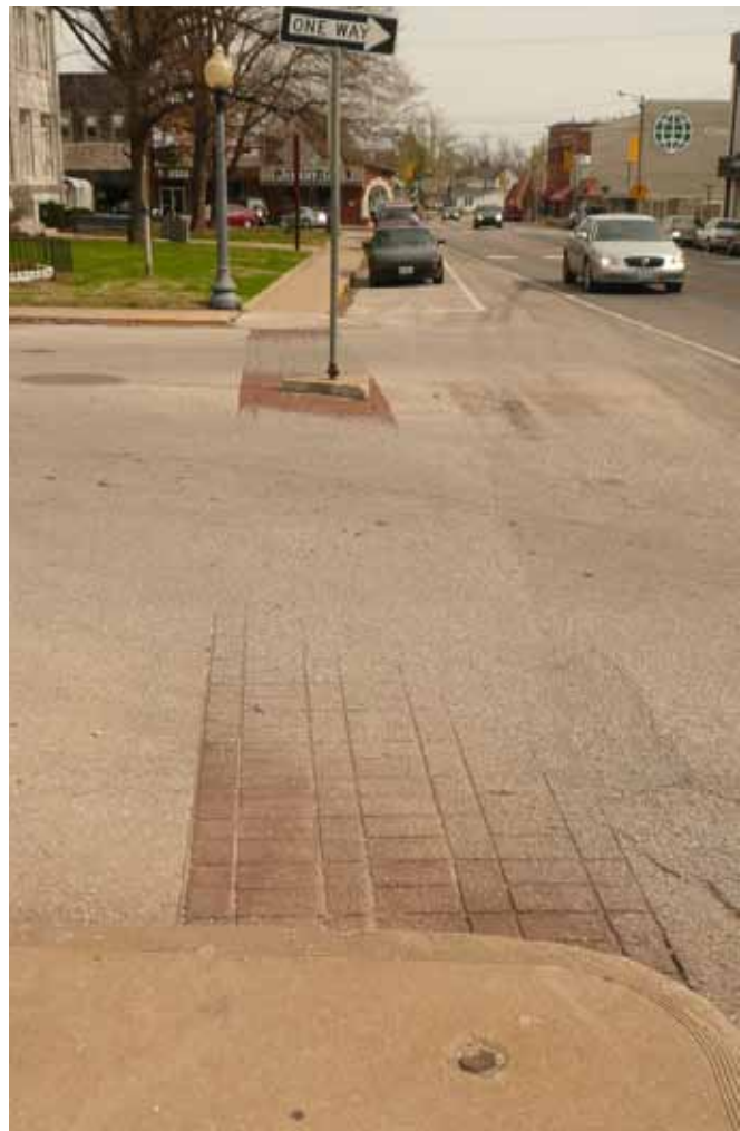
The crosswalk at the southeast corner of the courthouse does not provide a clear and unobstructed path for pedestrians.
