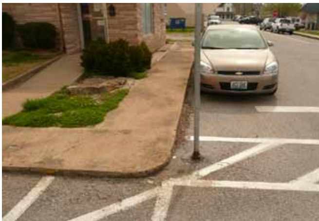
In many locations, there is no ramp from the sidewalk to the street and traffic signs block the crosswalk.
